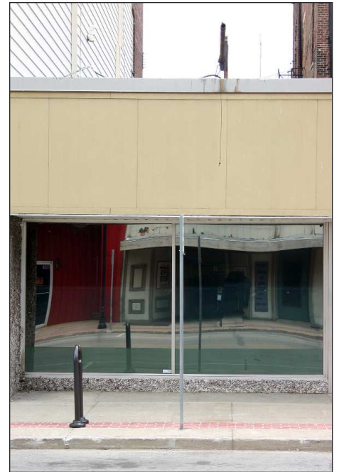
13 E. Market Street Retail Building 1 Story
