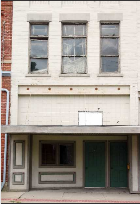
4 E. Market Street Retail Building 2 Story
