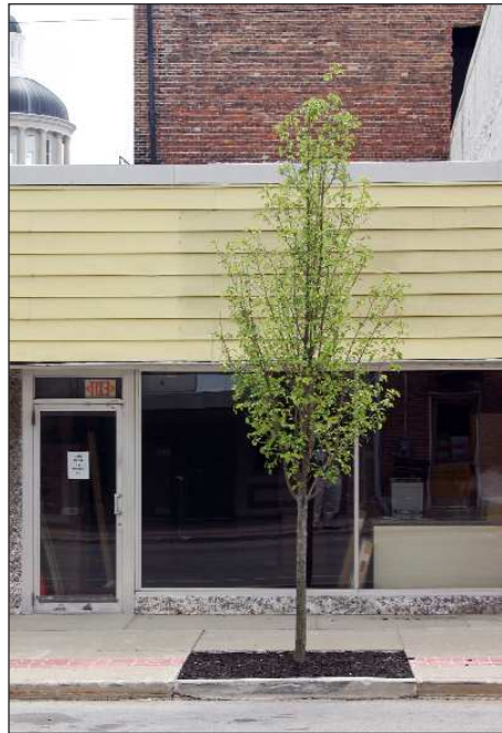
7 E. Market Street Retail Building 1 Story
