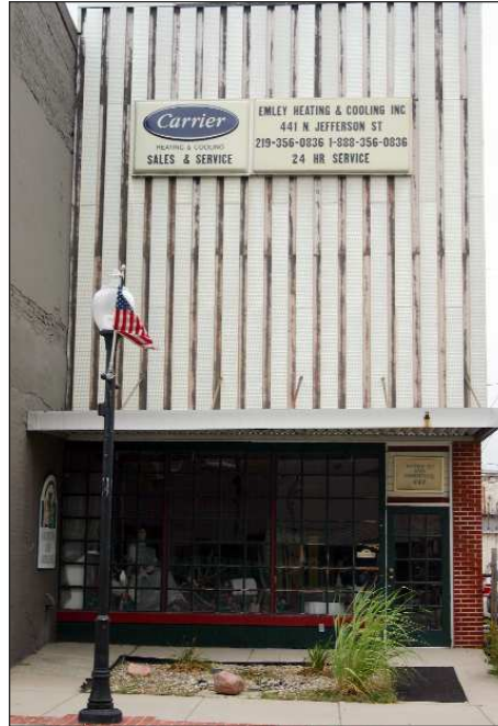
441 N. Jefferson Street Retail Building 2 Story
