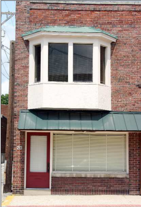
20 W. Washington Street Commercial Office Building 2 Story
