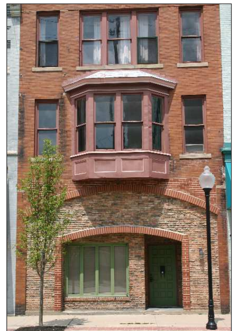
14 W. Market Street Residential/Retail Building 3 Story
