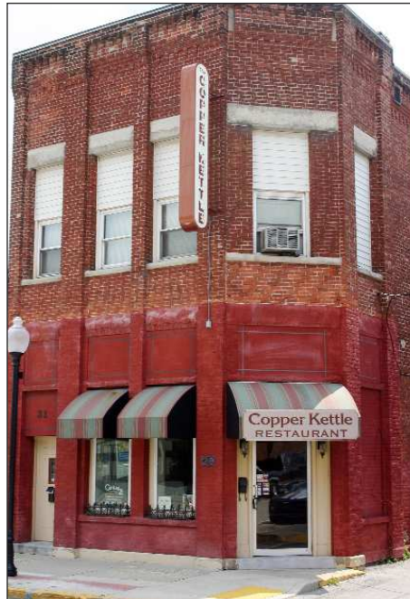
29 E. Washington Street Residential/Retail Building 2 Story
