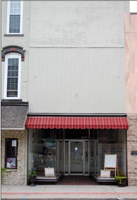
426 N. Jefferson Street Residential/Retail Building 3 Story
