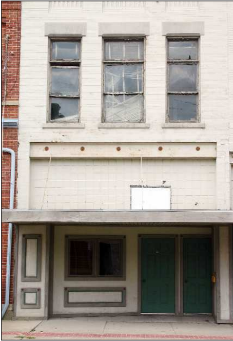
4 E. Market Street Retail Building 2 Story
