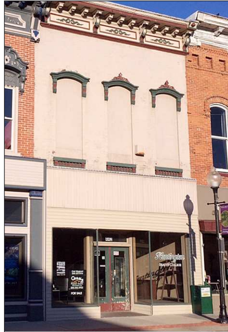
442 N. Jefferson Street Retail Building 2 Story
