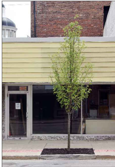
7 E. Market Street Retail Building 1 Story
