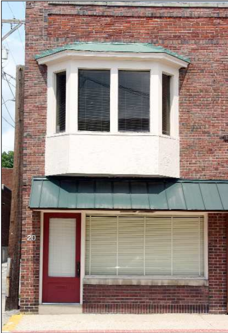
20 W. Washington Street Commercial Office Building 2 Story
